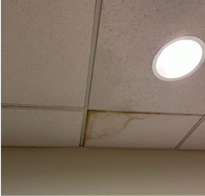
Board room ceiling
